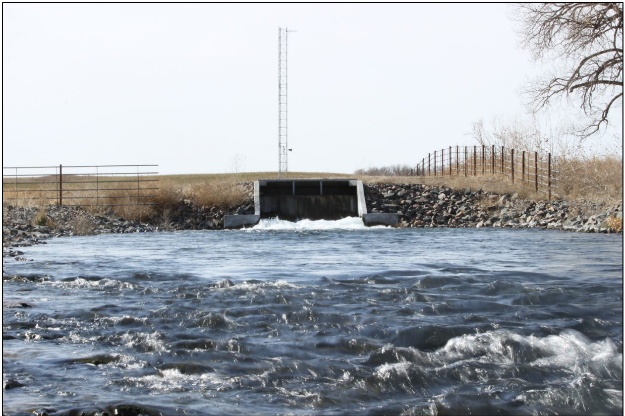
Figure 8. The South Discharge Pipeline of NCORPE on Medicine Creek; courtesy of N-CORPE
