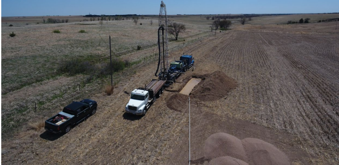
Figure 11. Construction of Flag Creek augmentation project
