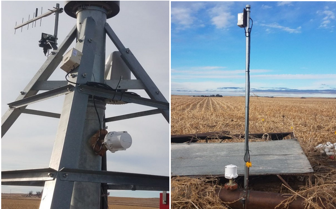
Figure 12. Two different mounting systems for Upper Republican NRD telemetry project.
