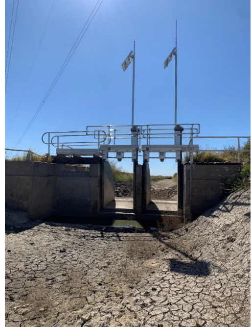
Figure 12. New Rubicon gates on canal operated by Frenchman-Cambridge Irrigation District.
