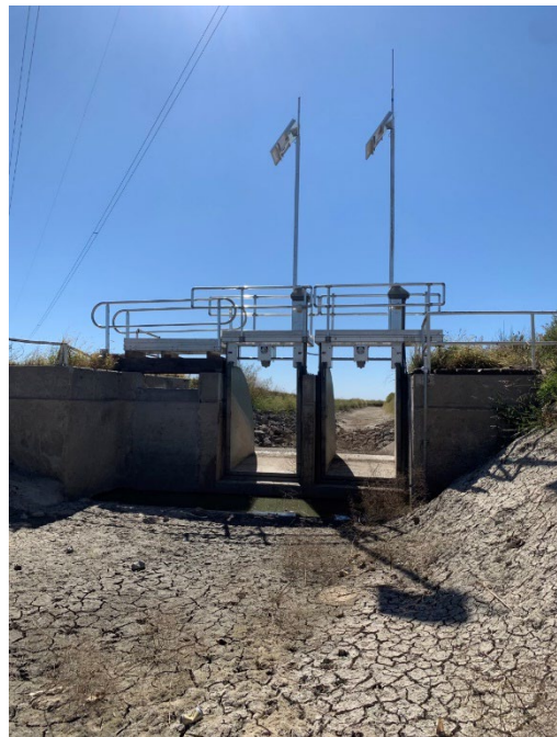
Figure 11. New Rubicon gates on canal operated by Frenchman-Cambridge Irrigation District.
