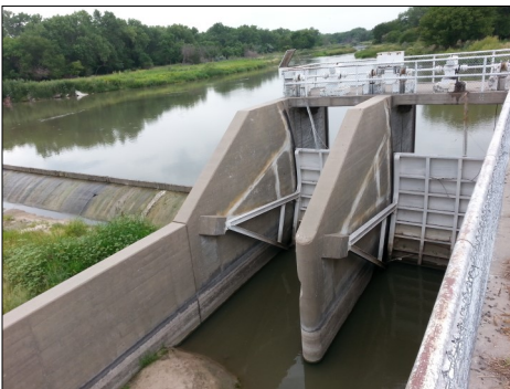
Diversion Dam on the Republican River
