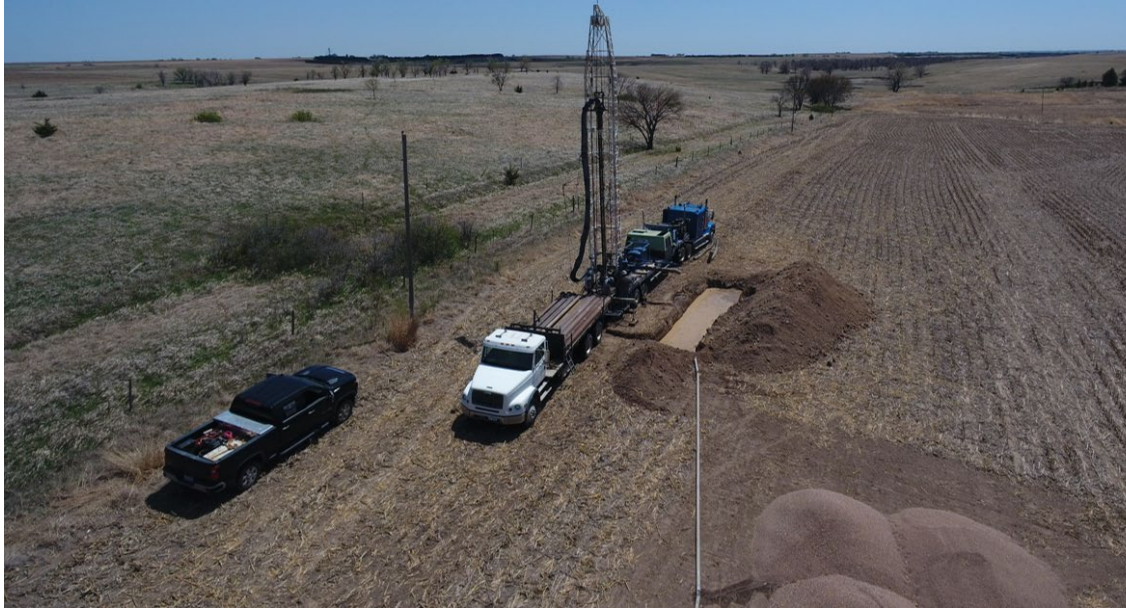
Figure 10. Construction of Flag Creek augmentation project
