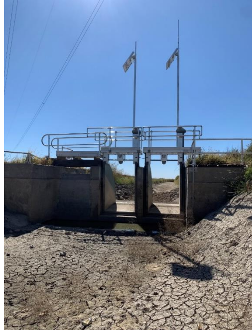
Figure 10. New Rubicon gates on canal operated by Frenchman-Cambridge Irrigation District.
