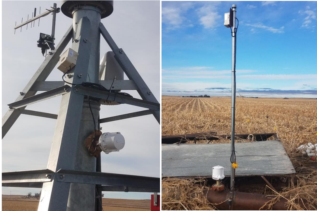
Figure 9. Two different mounting systems for Upper Republican NRD telemetry project.
