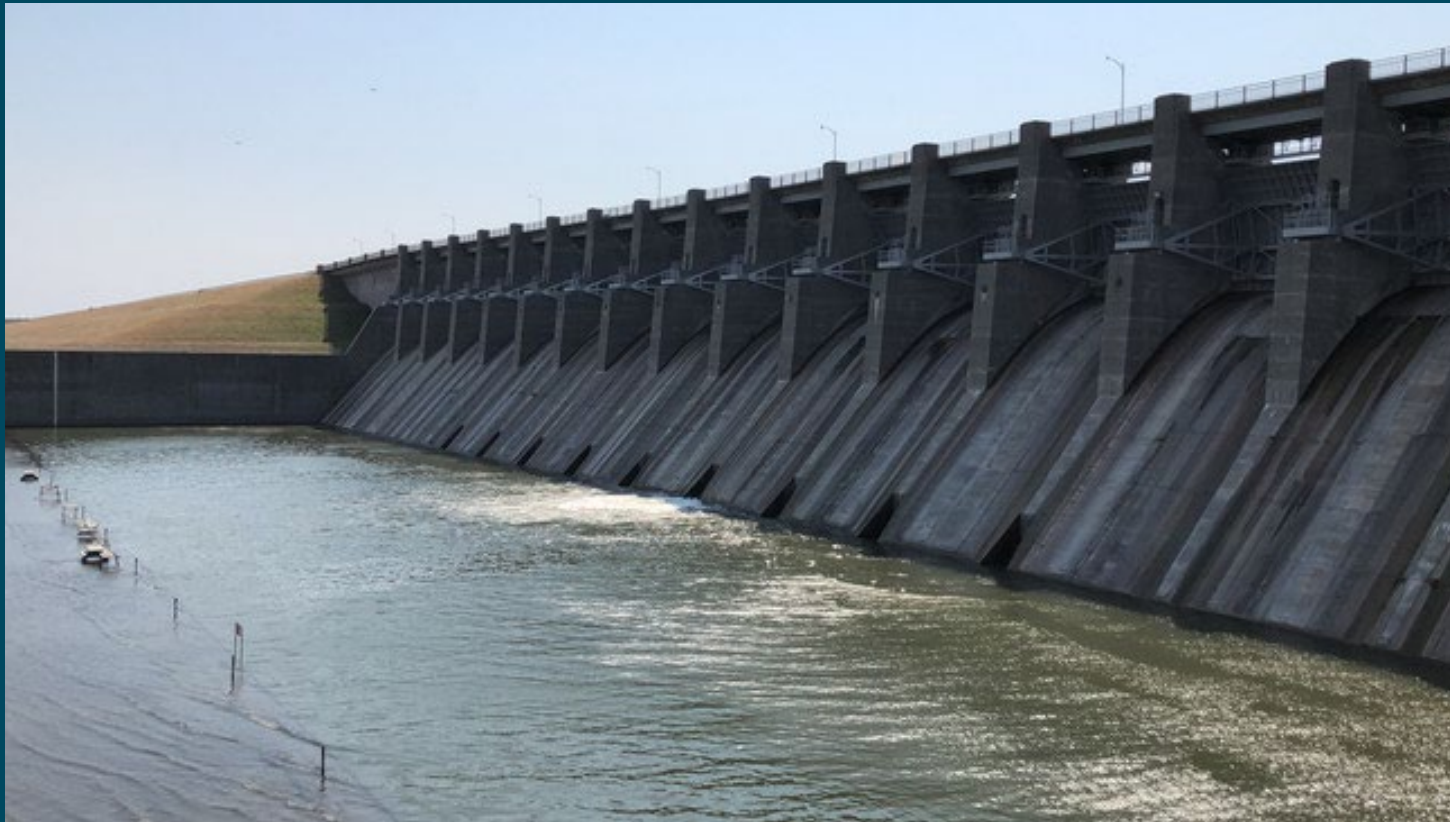
Harlan County Dam Spillway
